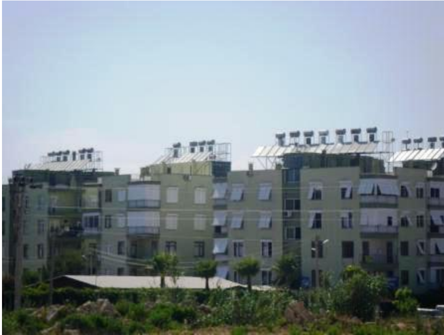
Rooftops in Antalya with ICS water heaters
